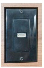
HDMI Connection (Located in a cabinet near TV) -Typical View
