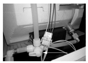
Water Heater Bypass Valve -Typical View (See "Water System Drain Valve Locations" chart at the end of this section for location on your model)
